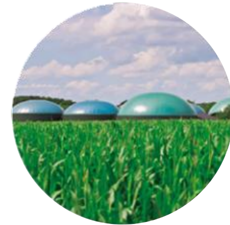
Energy from Chemical Fuels
