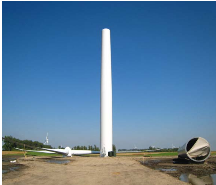
Figure 4-7 Partially constructed wind turbine tower
