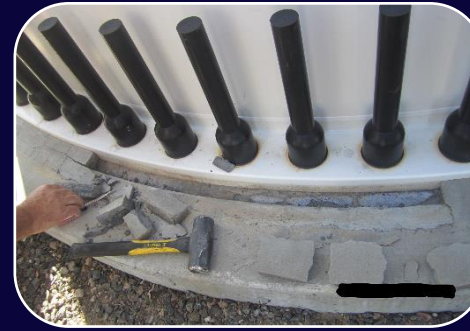
Grout failure
