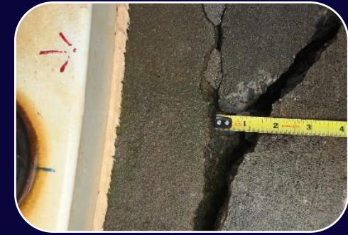
Concrete Cracking
