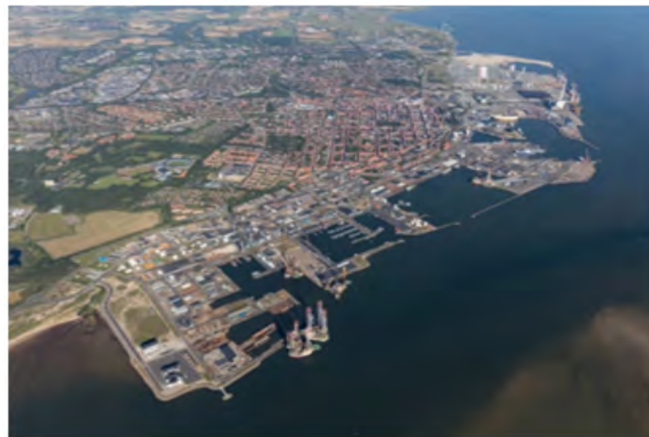
Exhibit 15: Port of Esbjerg
