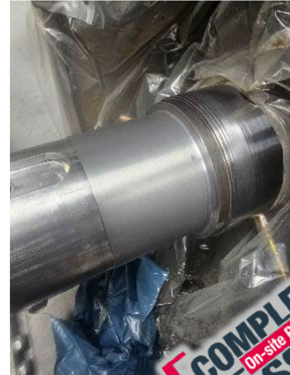
Recovered generator shaft after mounting of bush
